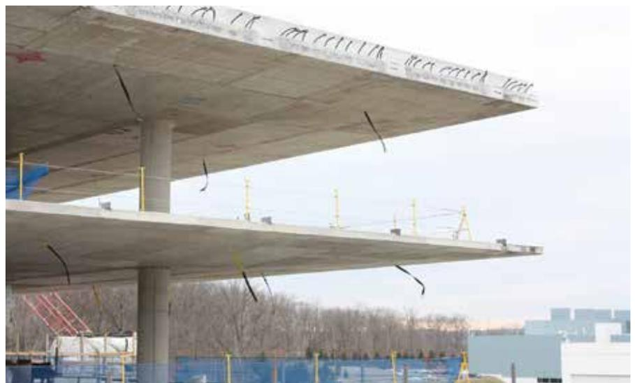
Fig. 5: View of 40 ft (12 m) cantilever at corners
