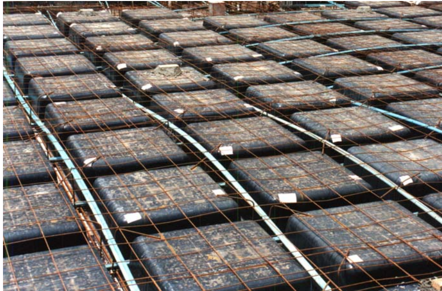
FIGURE 1-2 VIEW OF POST-TENSIONED WAFFLE SLAB CONSTRUCTION
