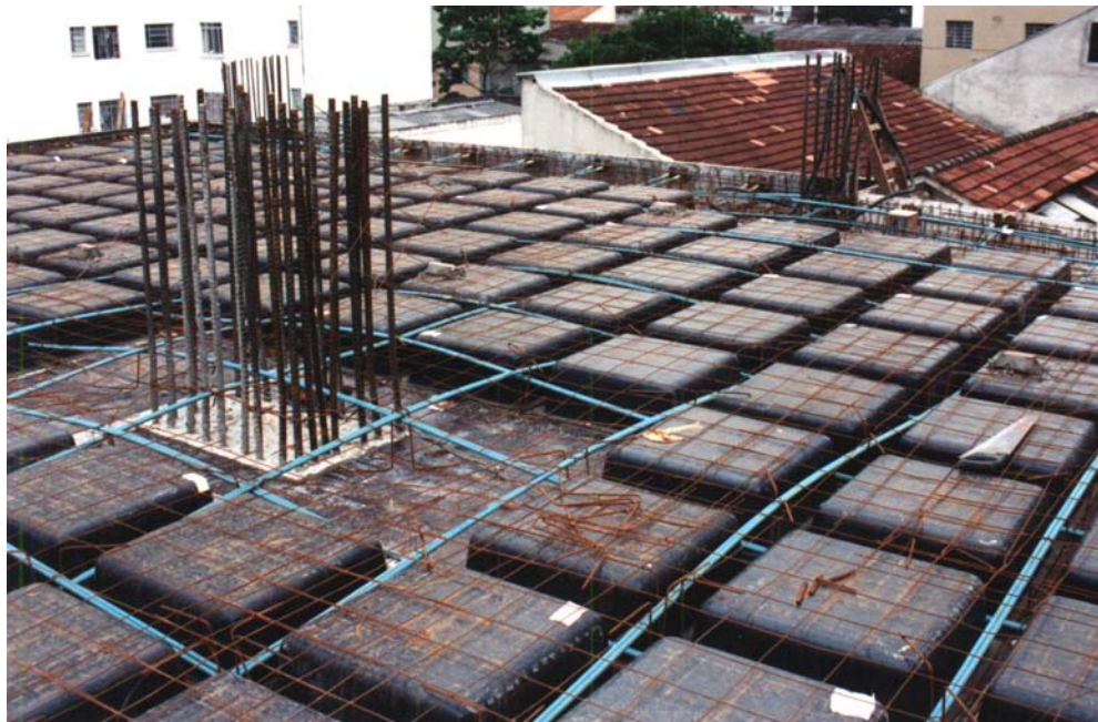
FIGURE 1-1 POST-TENSIONED WAFFLE SLAB CONSTRUCTION
